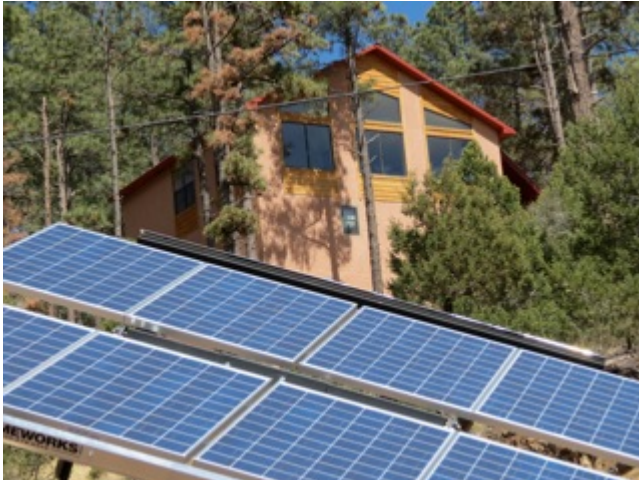
Photos of the: 11-kW grid-interconnected, single-axis tracking, and pole-mounted solar photovoltaic system to generate electricity used by the Sun Valley Water and Sanitation District in Alto, N.M.
