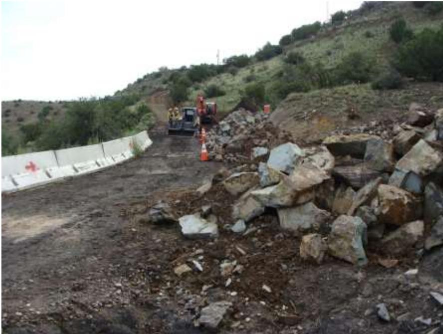
*Rock waiting to be placed in channels. The temporary Jersey barriers on the left are being replaced with architectural precast concrete units.*
