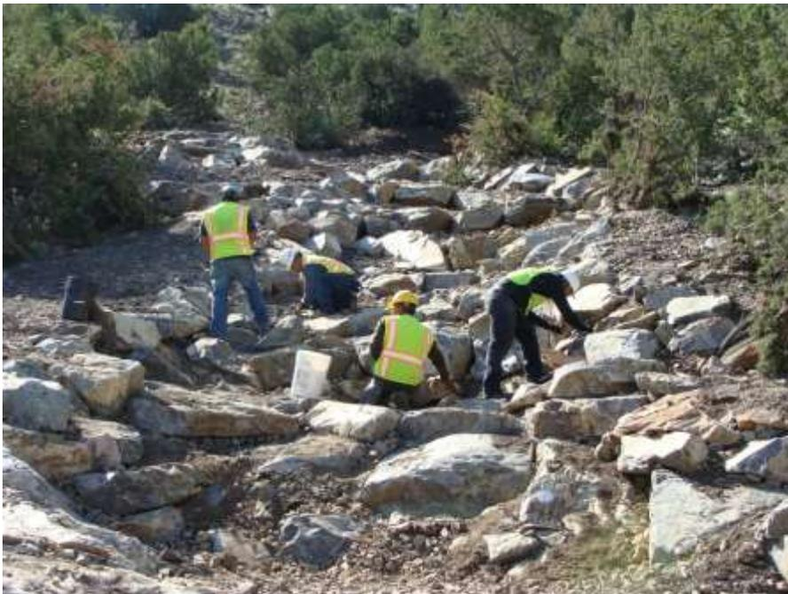
*Hand fitting small rock into a large rock drop structure*
