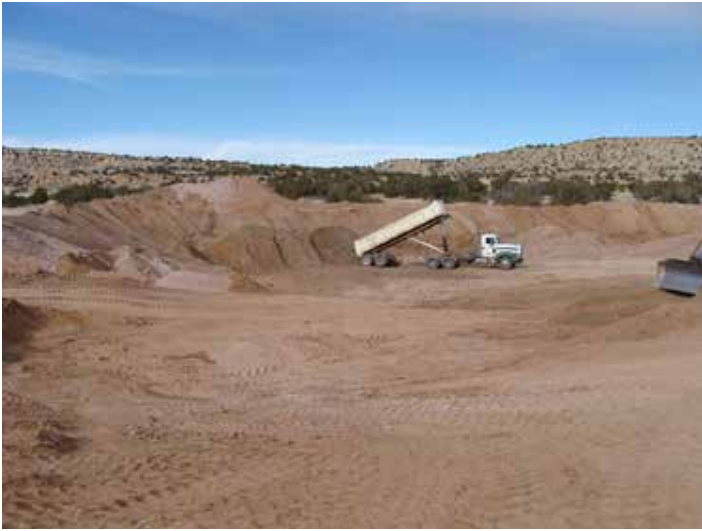
Dumping radioactive mine wastes into the Grants Phase III Repository
