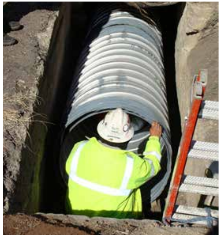
Madrid - Slipline pipe being placed in old box culvert
