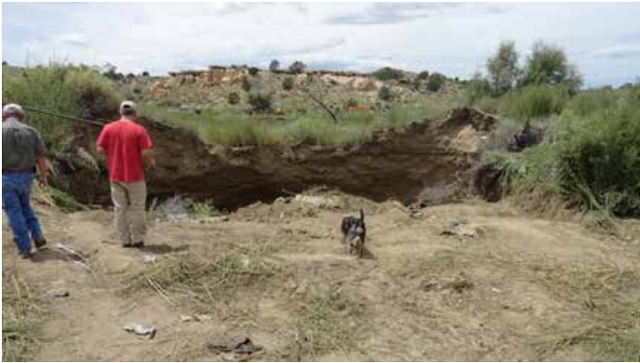
Allison Mine sinkhole, August 2015
