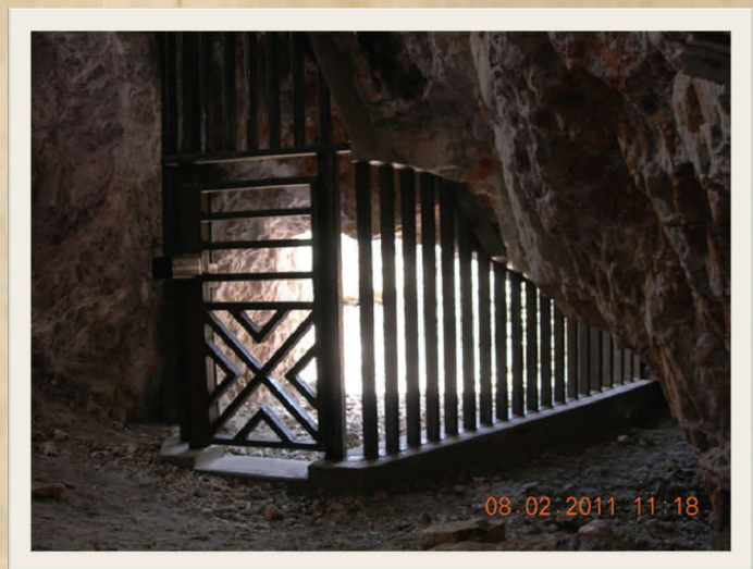
Adit #1 after Construction (Feb. 2012 left and Aug. 2011 right) (Note the bat compatible horizontal openings in the hinged door)
