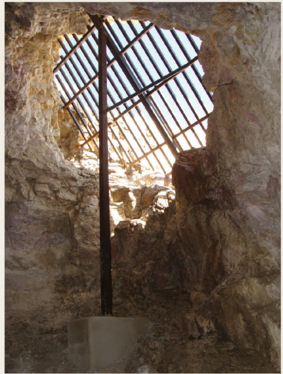
Stope #1 after Construction (Aug. 2011)
