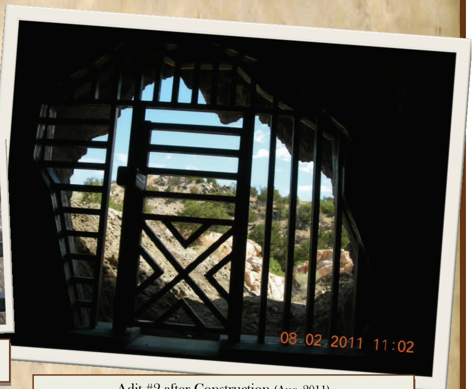
Adit #2 after Construction (Aug. 2011) (Note bat compatible openings and unlocking mechanism at hinged door)
