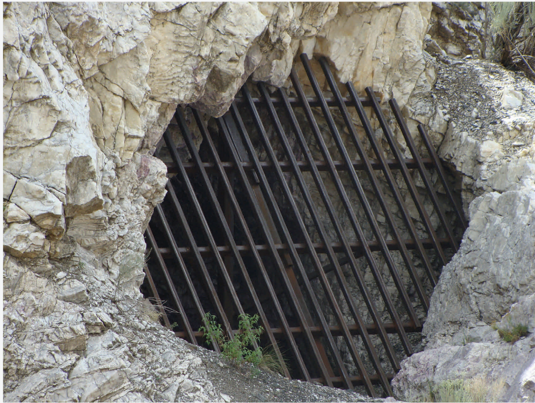
Stope #1 Closure at the Harding Pegmatite Mine (Aug. 2012)
