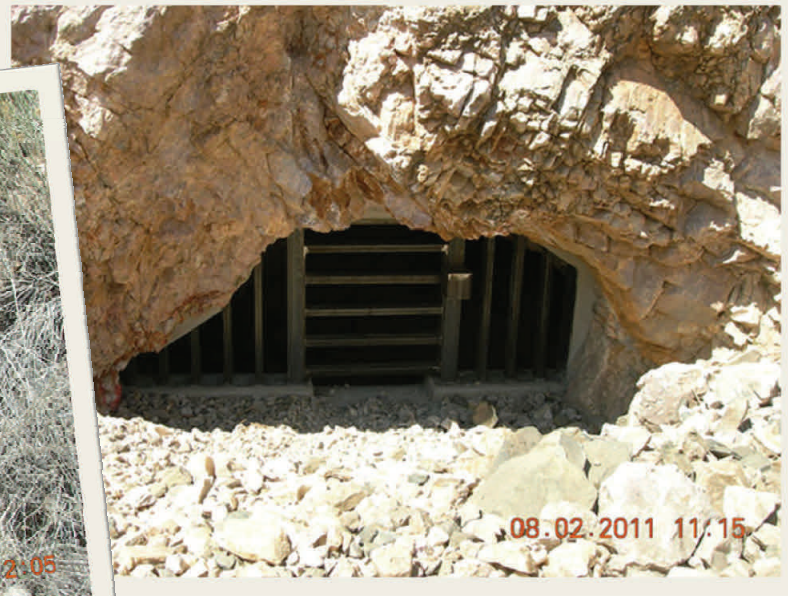
Adit #5 after Construction (Aug. 2011) (With bat compatible openings in hinged door)
