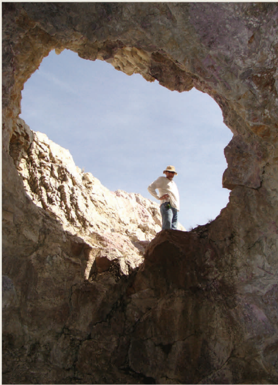
Stope #1 before Construction (Apr. 2010)
