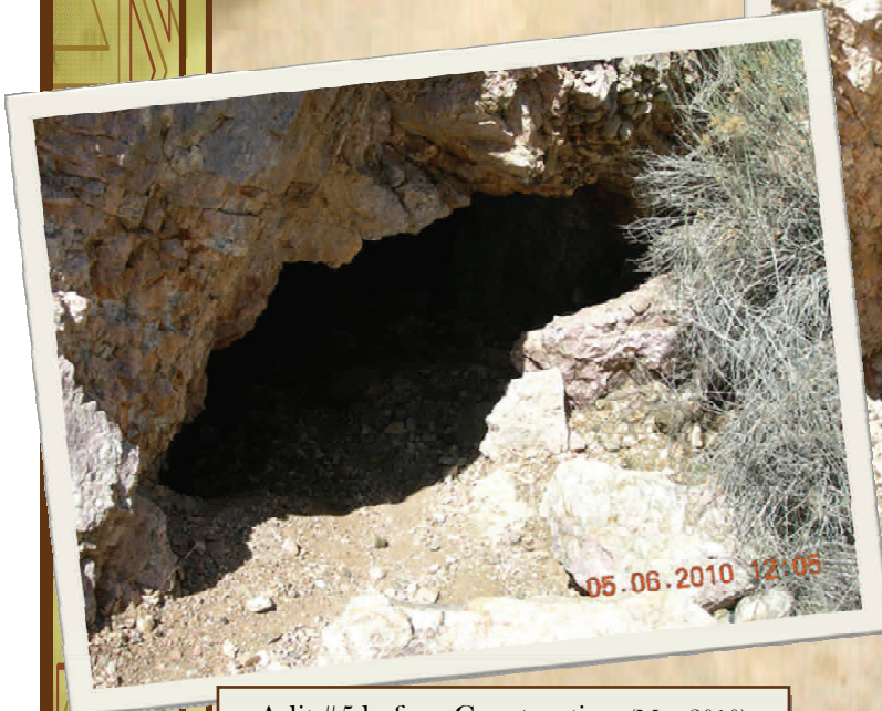
Adit #5 before Construction (May 2010)
