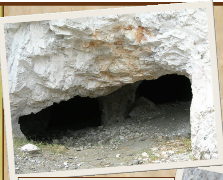
Adit #1 before Construction (Aug. 2009)
