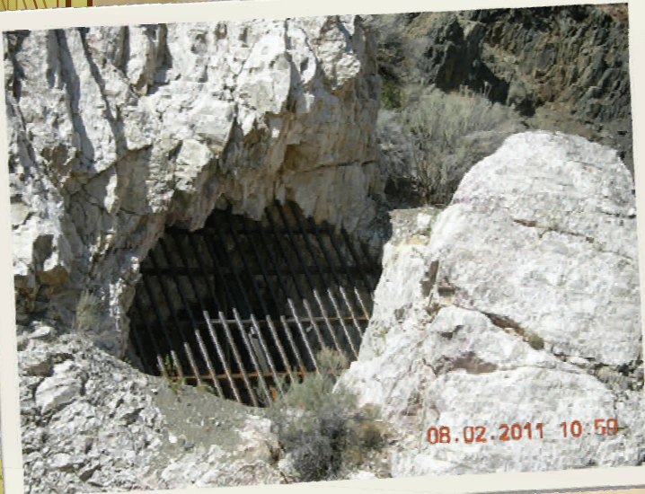
Stope #1 after Construction (Aug. 2011)
