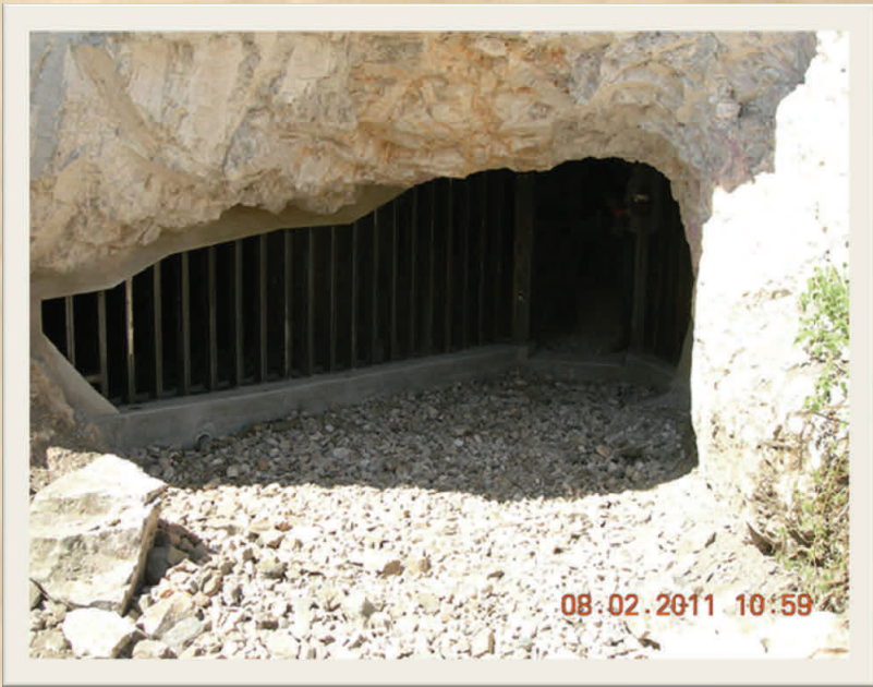
Adit #1 after Construction (Aug. 2011)
