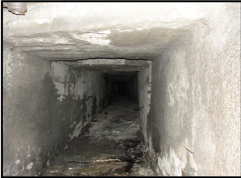
Figure 24. Box culvert after jet flushing, February 2015. Note exposed tree roots on floor.
