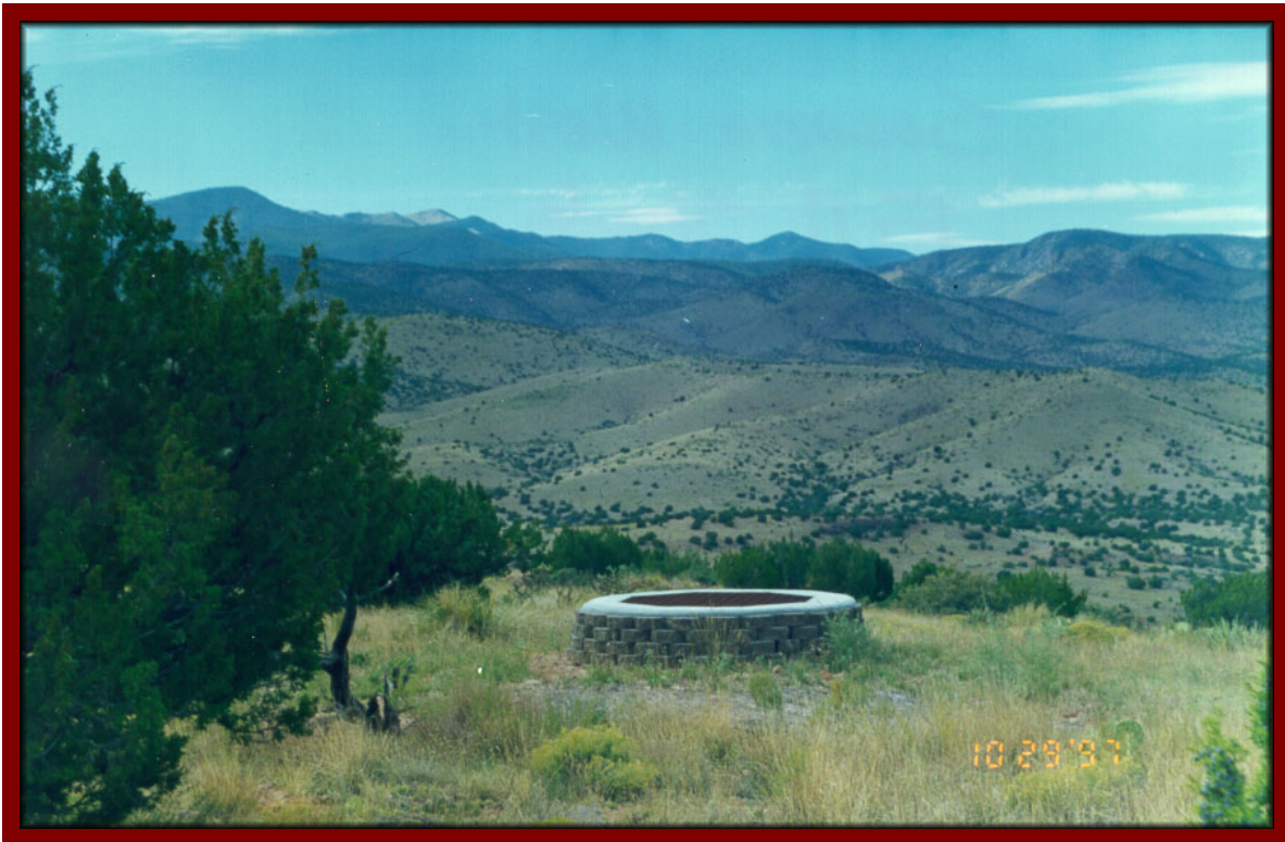
Completed grated closure at the Feature 11 Shaft one year after construction
