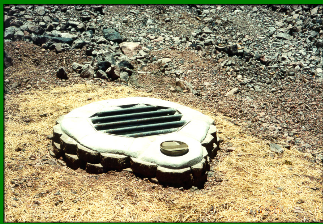
Completed bat closure with corrugated steel pipe riser at the Feature 15 Shaft
