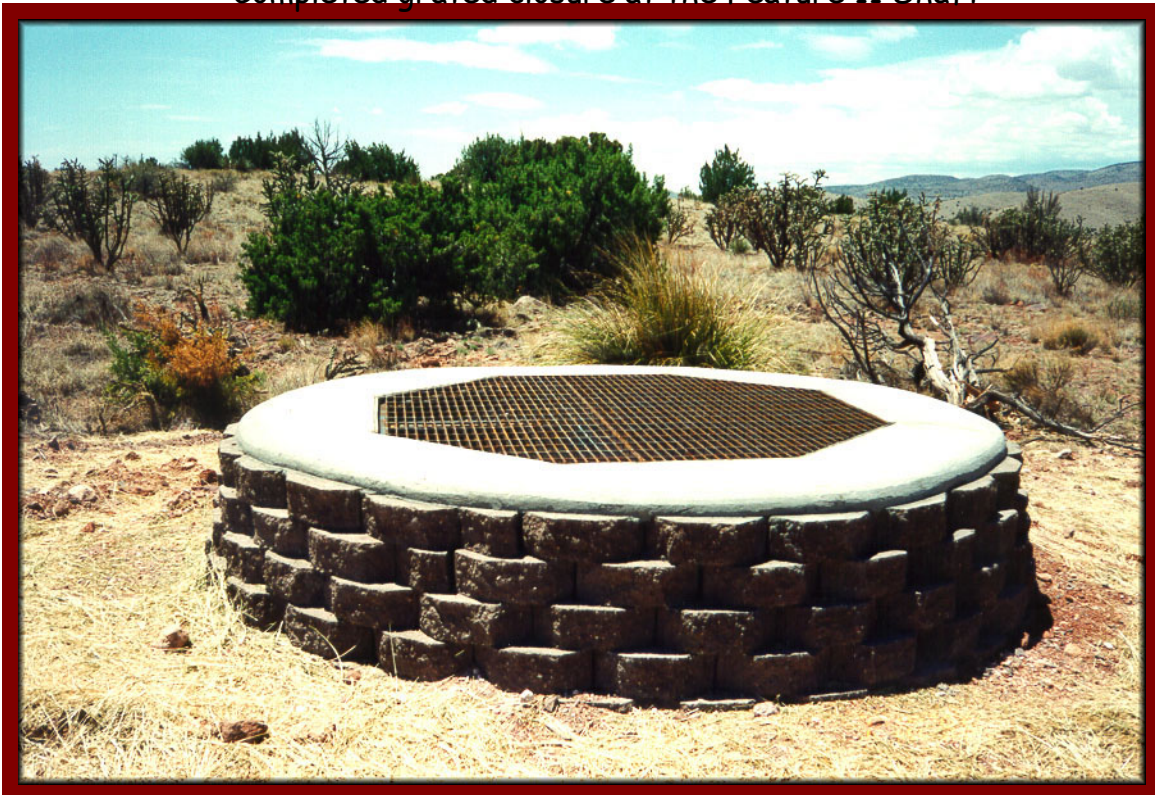
Completed grated closure at the Feature 11 Shaft
