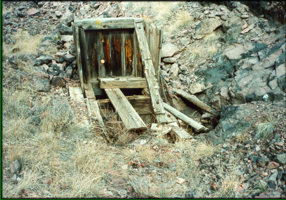
Feature 15 Shaft, preconstruction
