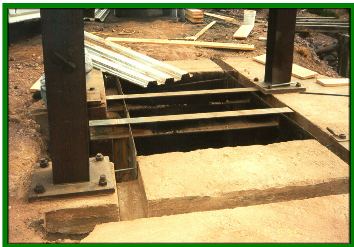
Collar at the Feature 4 Shaft cleaned and ready for form construction
