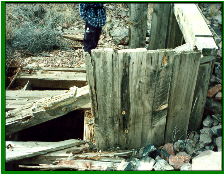
Feature 15 Shaft, preconstruction
