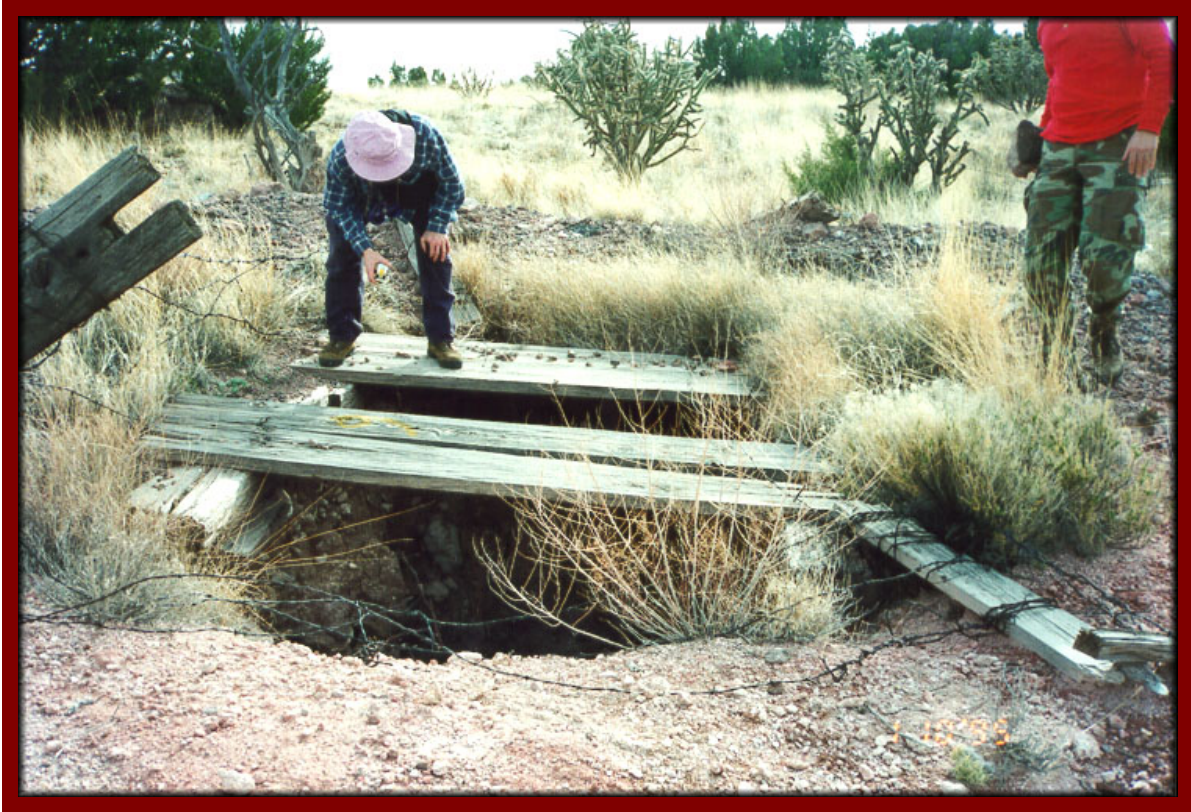
Feature 11 Shaft, preconstruction
