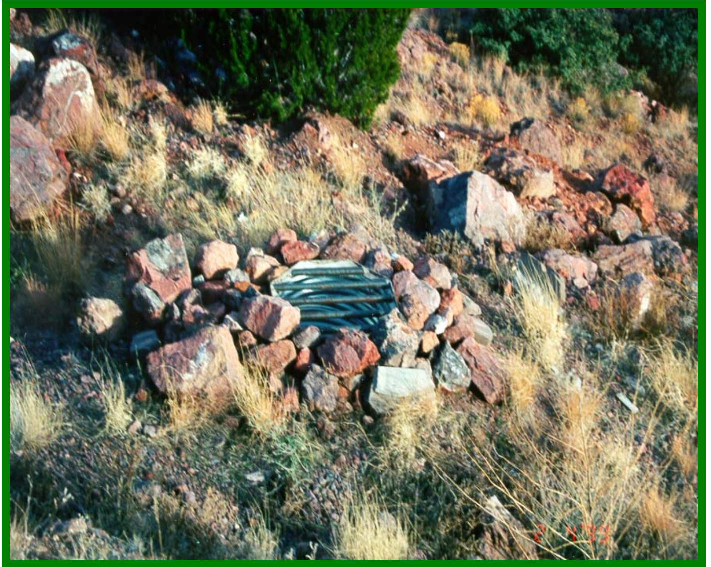
Feature 18 bat closure following vandalism, mortarless concrete units replaced with native rock
