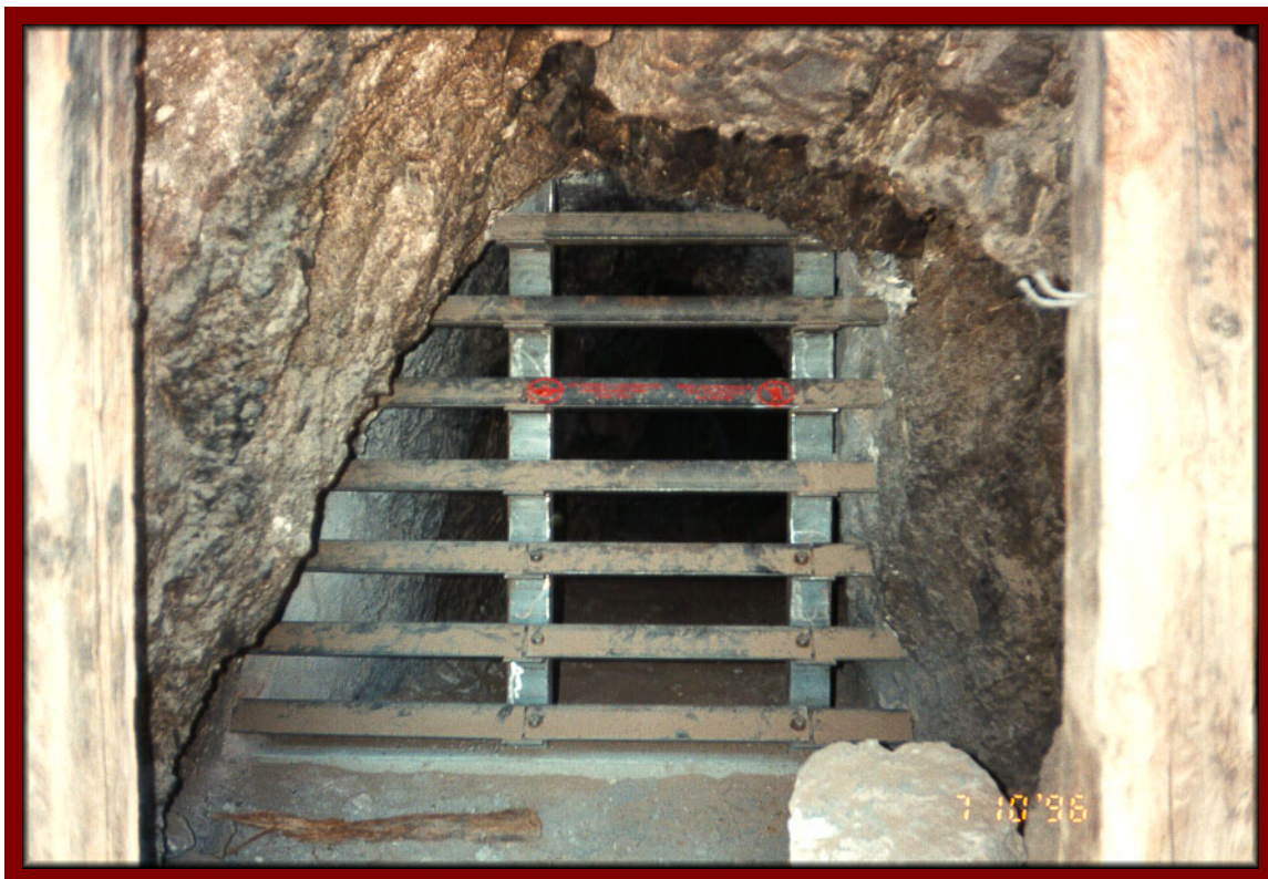
Completed bat closure in the Feature 7 Adit
