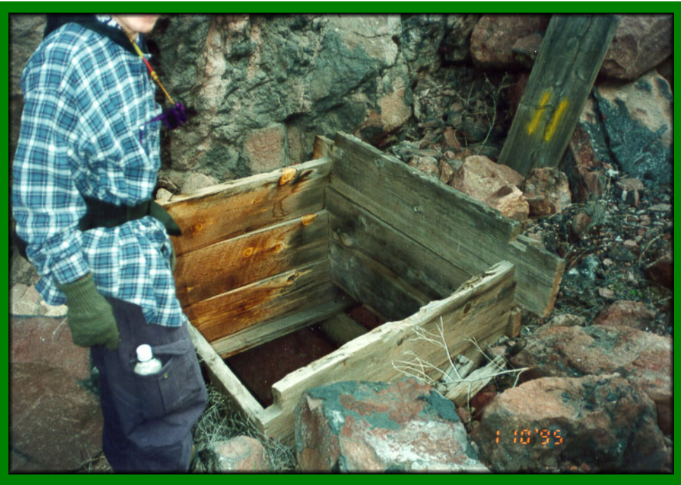
Feature 13 Open Stope, preconstruction
