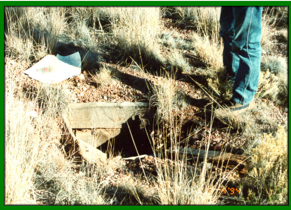
Feature 18A Vent Shaft, preconstruction
