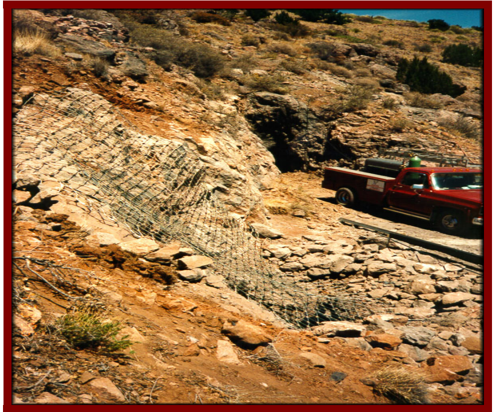
Completed cable net at Feature 6A Shaft
