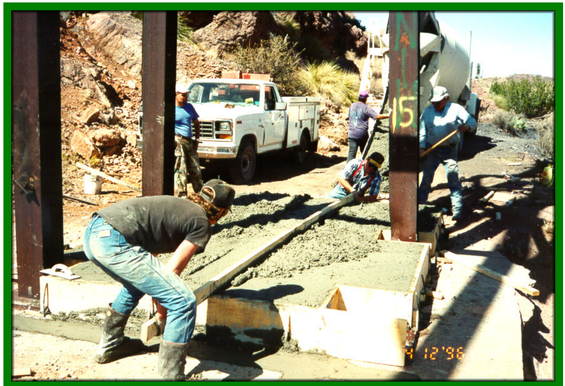
Placing concrete at the reinforced concrete slab at the Feature 4 Shaft
