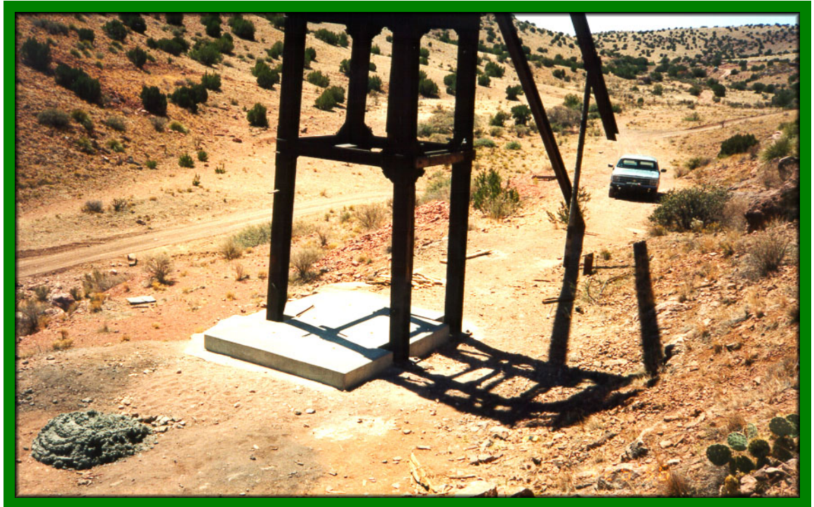
Newly completed concrete slab at the Feature 4 Shaft
