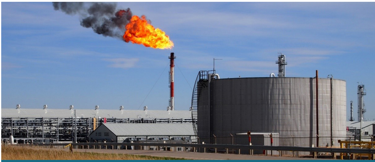
FIGURE 2. Natural gas being flared at the Hess Corporation gas plant in Tioga, North Dakota, due to maintenance issues. Photo credit Amy Dalrymple / Forum News Service (Source) 2
