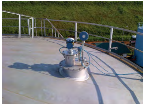
Figure 3.4: Manways are normally located near the tank wall which provides mechanical stability.
