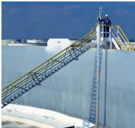
Figure 3.1: Still-pipe in an open floating roof crude oil tank.
