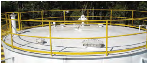
Figure 2.14: Fixed roof tank openings.
