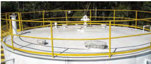
Figure 2.14: Fixed roof tank openings.
