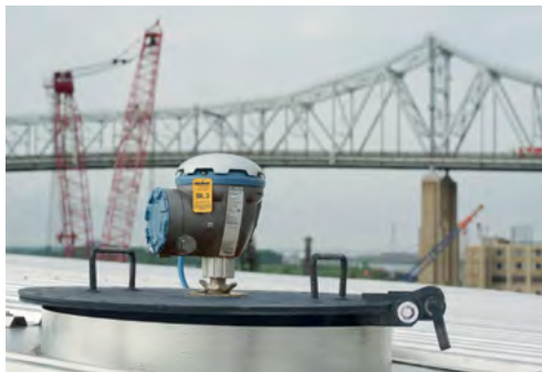
Figure 2.10: Modern radar level gauge on a fixed roof tank.
