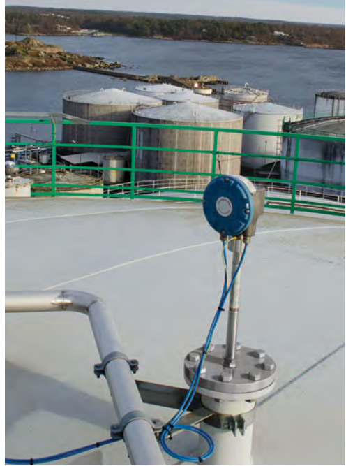
Figure 6.1: Top mounted temperature transmitter for up to 16 spot temperature elements.
