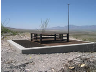
This cupola closure allows for use by owls and possibly bats. The lack of backfill material nearby made this a sensible option.
