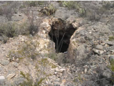
Adit that leads into the interior workings of the mountain. AML had to remove a colony of africanized bees at the entrance before starting construction.
