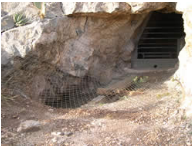
This bat gate was built to allow bats to come and go while keeping curious humans out. The stope at the front entrance, which is not used by bats, was covered with high-tensile steel mesh.
