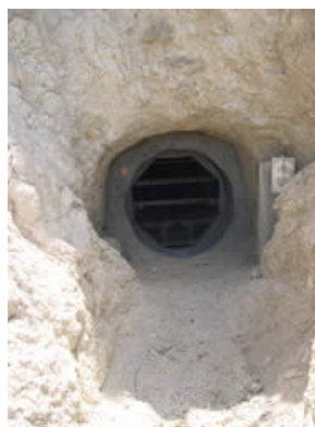
The bat gate was built to allow bats to come and go while keeping curious humans out.
