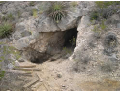
An adit with an open stope near the entrance. The stope was not used by bats and was covered with high tensile steel mesh. The bat gate was built just inside the view of this photo angle.
