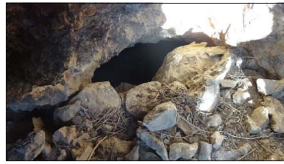
INNER ADIT TO BE MUCKED OPEN
