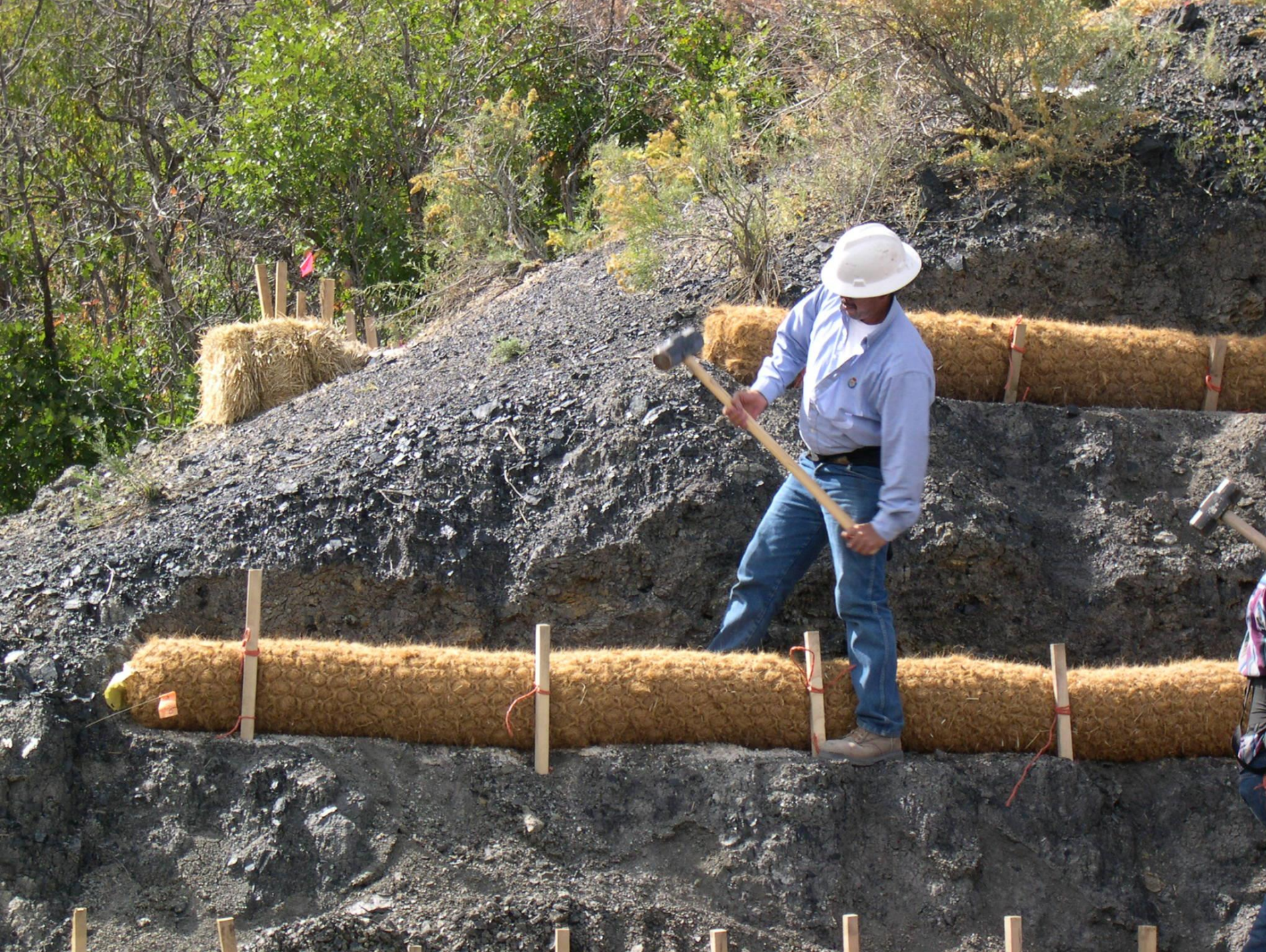
Example: AML Sugarite Gob Reclamation Project – BEFORE
