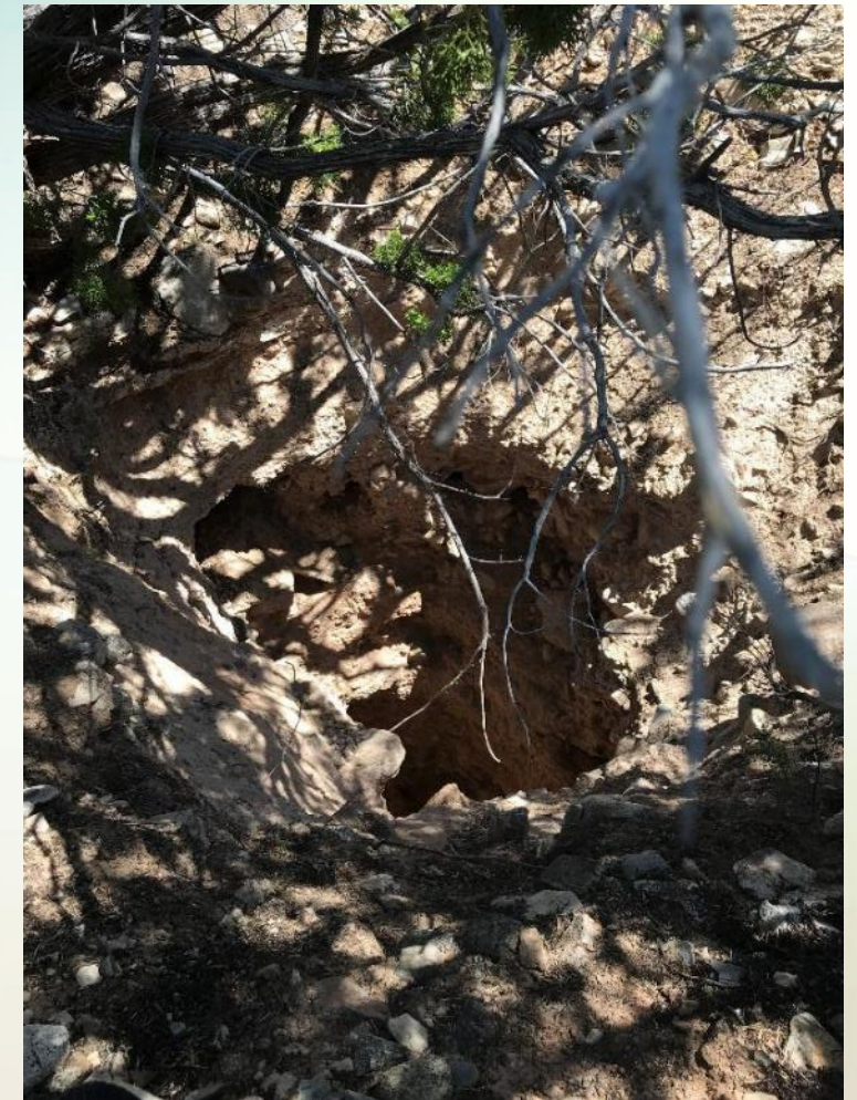
Shaft G-23: 4.5' WIDE BY 5' LONG SHAFT IN INTERIOR OF FEATURE WIDENING TO 10.5 WIDE BY 11' LONG PIT. FEATURE IS 14' DEEP FROM TOP OF PIT.
