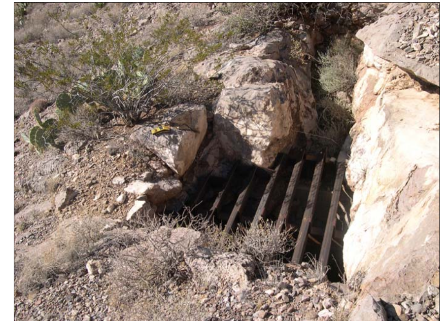
EXAMPLE PHOTO OF COMPLETED HORIZONTAL BAT GATE (GAGE MINE SAFEGUARD PROJECT)
