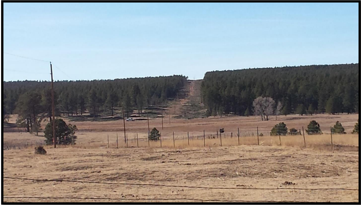
Image 3 Hillside showing power line fuels reduction treatment. Image courtesy of NM State Forestry.
