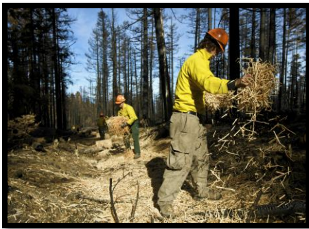
Image 6 Spreading mulch to reduce post-fire erosion
