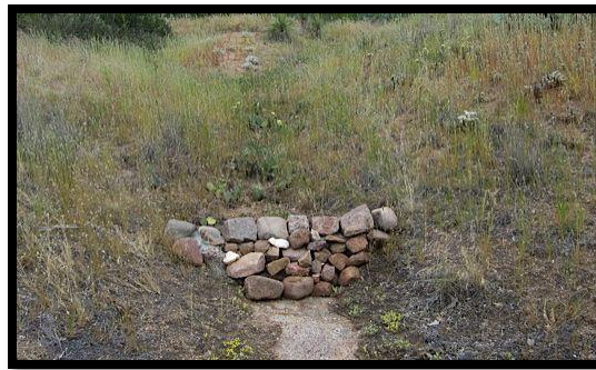
Image 3 a check dam stabilizes soil behind it
